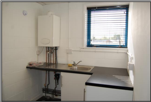
First Floor Kitchen
